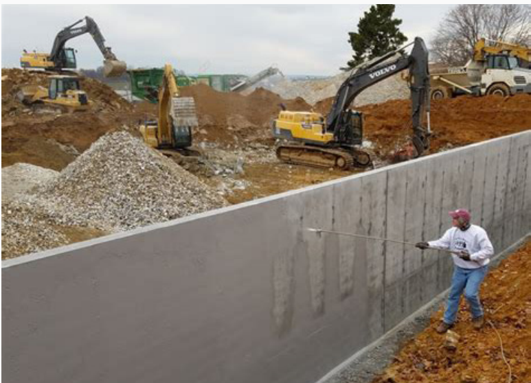
FIGURE 12 (a) Various forms of flood mitigation, (b) Spray on waterproof layer for wall protection
