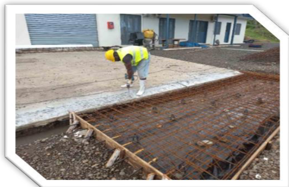
Figure 2: Nabouwalu NFA Office
